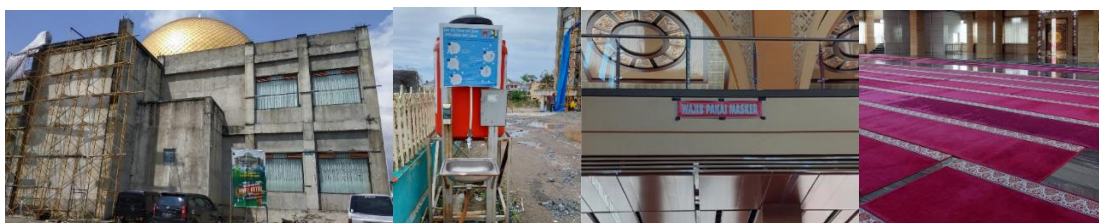
Figure 1. The Facade of the Jami' Aur Kuning Mosque, Handwashing Area, a Mandatory Sign of Wearing a Mask, and Prayer Area
