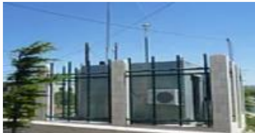
Figure 5: One of Amman's monitoring stations
